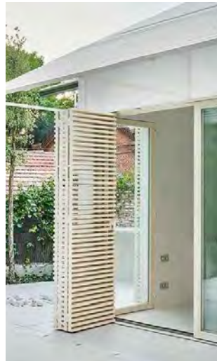
TM:01 LIGHT COLOURED TIMBER SHUTTERS
